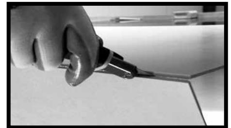
**Fig.12** - As far as SLIMTECH 3plus and SLIMTECH 5plus are concerned, after engraving the ceramic part and splitting the slab, complete the operation by cutting the fiberglass mesh with a standard cutter.
