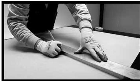
**Fig.10** - To ensure that the engraving is as straight as possible, you may use aluminum levelling rods of the type commonly used by brick layers.
