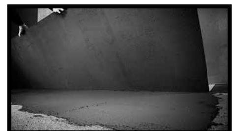
**Fig.68 - 2** - Rest the slab on its long side and guide it towards the floor.
