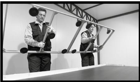
**Fig.4/5** - All versions of SLIMTECH slabs, of size 300x100 cm, can be handled by two persons, using a special frame. Fasten the frame to the slab when it is still on the pallet. Now raise the frame and slab to eliminate the suction effect.
