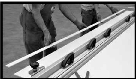
**Fig.13** - A practical tool for cutting is the tile cutter ruler (for instance Keracut from **Sigma** or Free-cut from **Raimondi**). As far as SLIMTECH 3plus and SLIMTECH 5plus are concerned, after engraving the ceramic part and splitting the slab, complete the operation by cutting the fiberglass mesh with a standard cutter (**Fig.12**).
